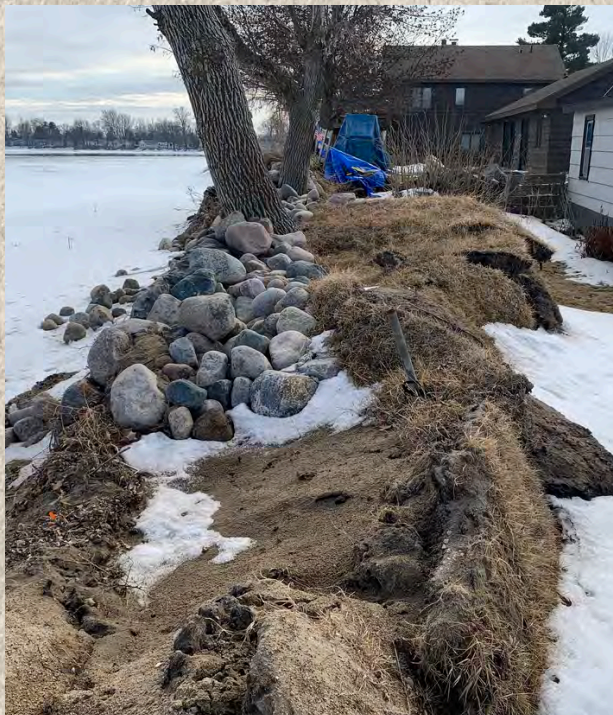
Riprap will not defend against ice damage.
